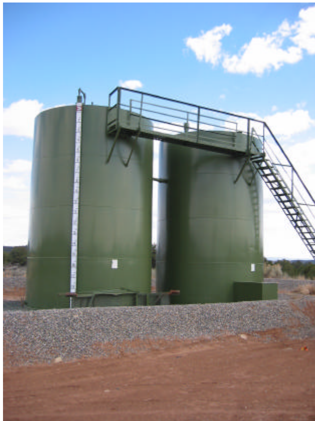
Figure 12: Produced Water Storage, Allison Unit Production Well
