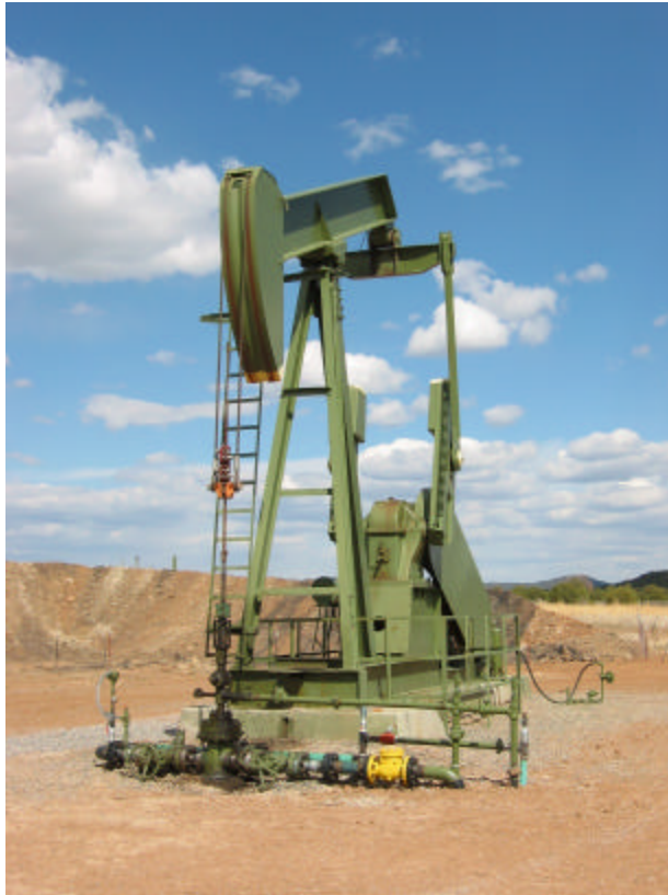
Figure 9: Typical Production Well Surface Configuration, Allison Unit
